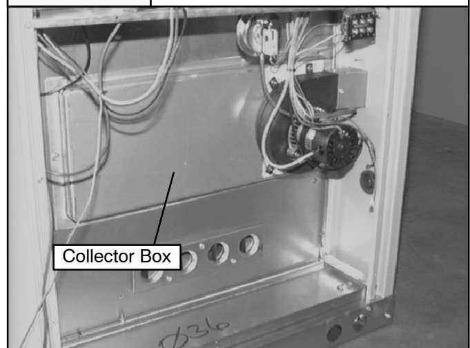
Burners, Valve, and Burner Box Removed
