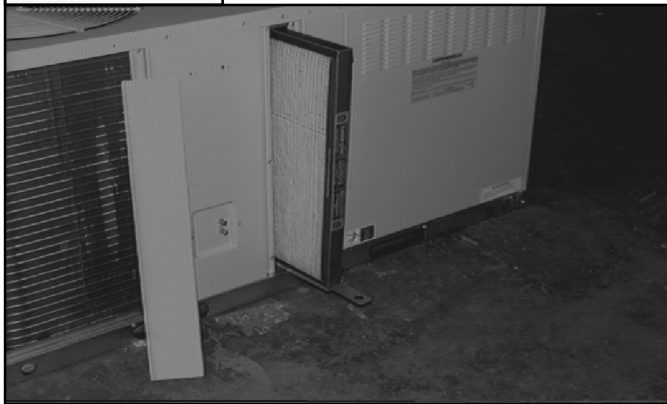
Figure 40 Access to Built-In Filters
