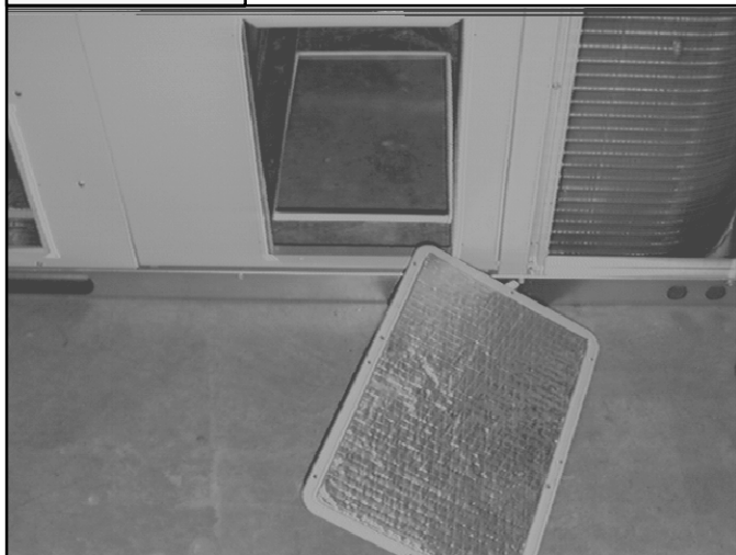
Blockoff Plate Removed (Return Air Compartment)
