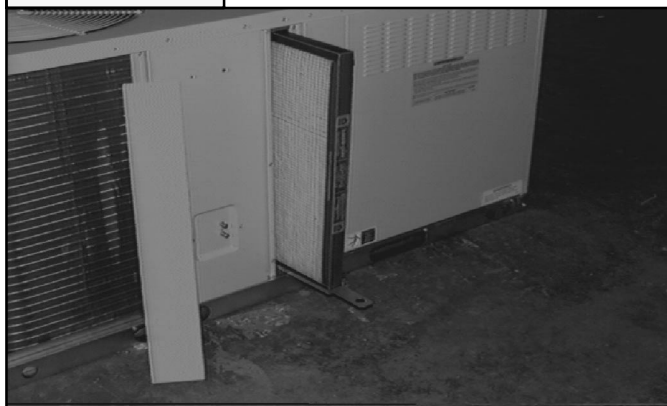
Access to Built-In Filters (Except "B" Chassis)
