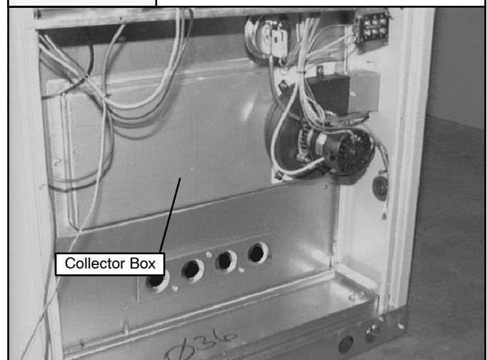
Burner Assembly Removed
