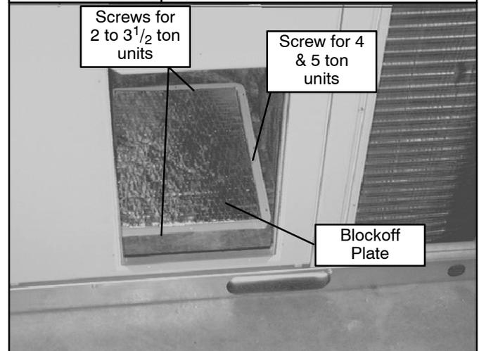
**FIGURE 7** Blockoff Plate Removed (Return Air Compartment)
