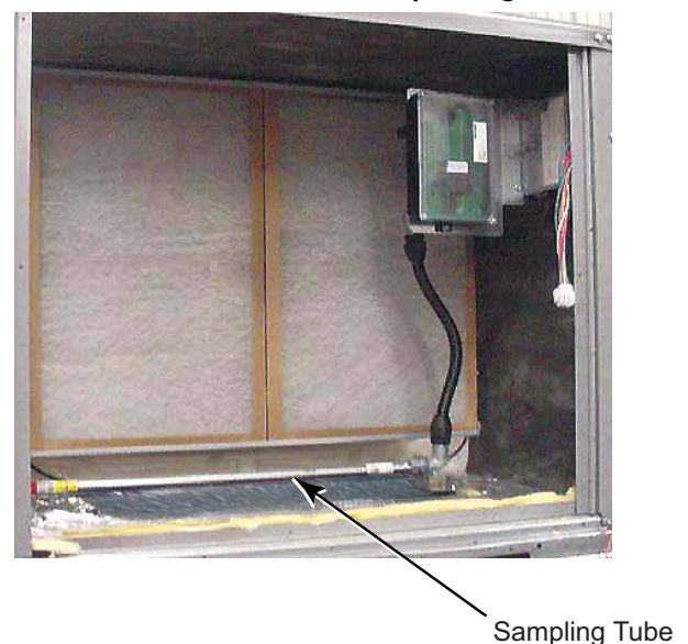
FIGURE 35 Return Air Sensor Operating Position
