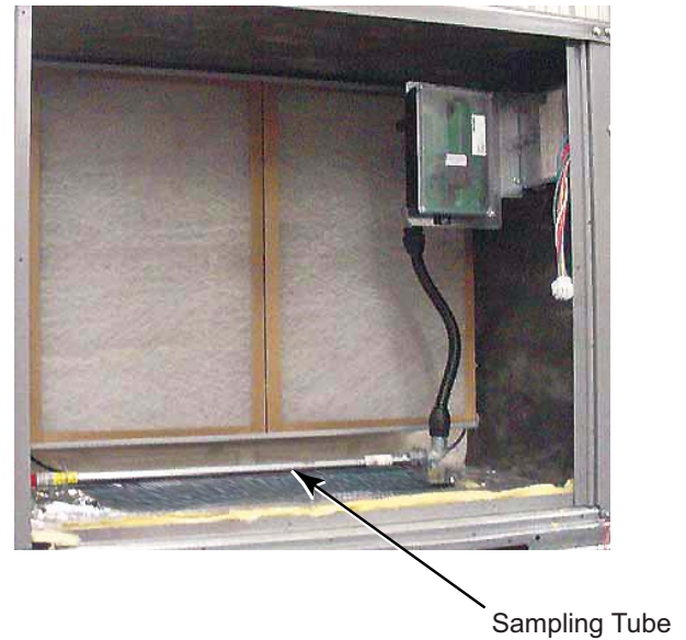
FIGURE 40 Return Air Sensor Operating Position
